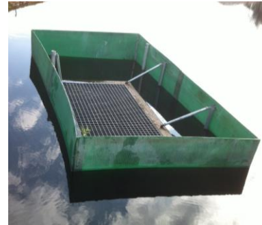
2014 Pic with New Grate
